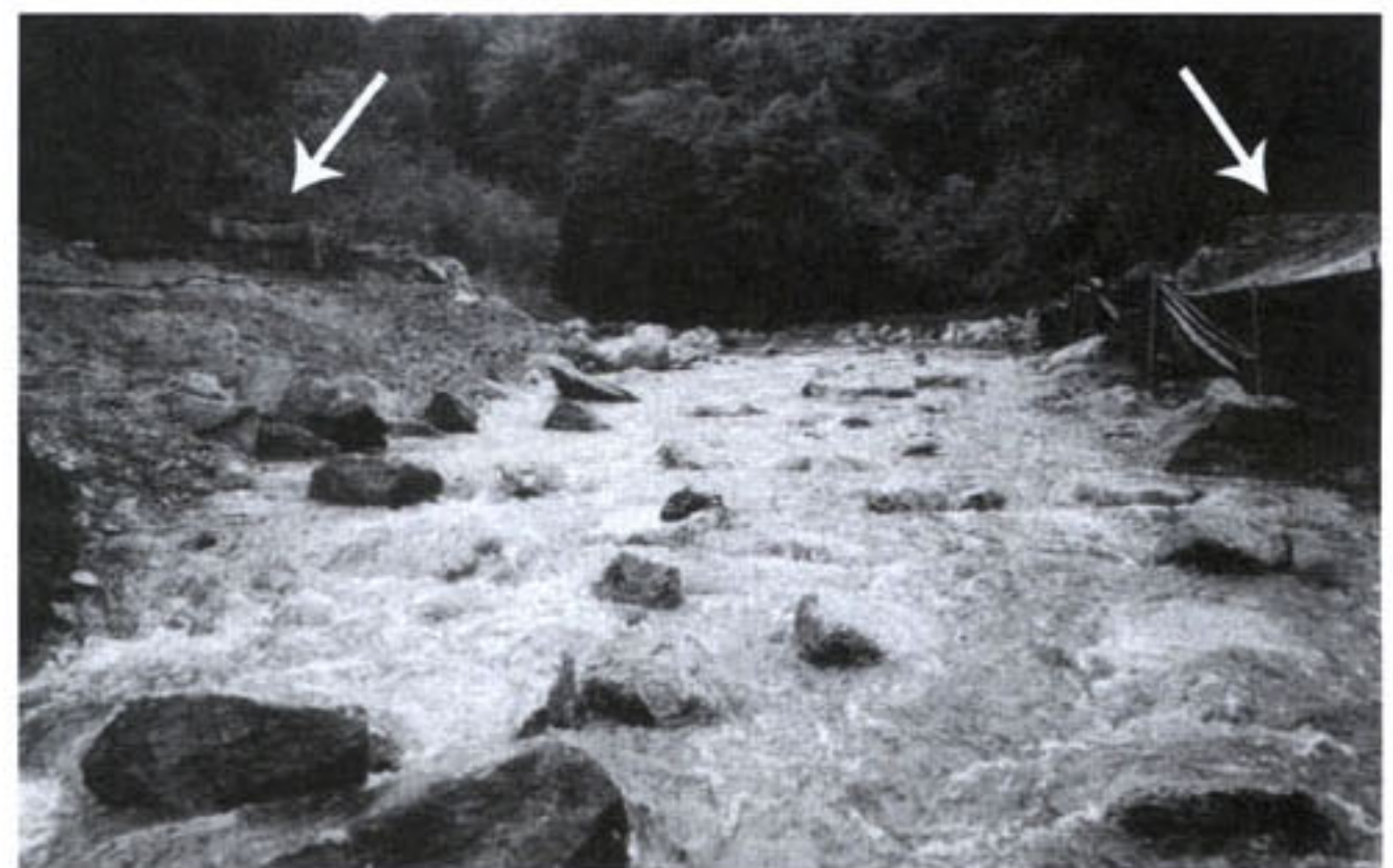
Figure 2. Example of a dam removal approximately one week following removal. View is facing upstream from within the area of the removed dam. White arrows mark the remaining abutments of the original dam face. The channel has been created by removing impounded sediment to match the shape of a downstream reference reach. Cobble substrate placed on the streambed will resist erosion in accordance with sediment transport theory. The banks are cut to a stable slope, stabilized at the base with large cobbles, and seeded with native vegetation. Compare with the channel in figure 1b.
