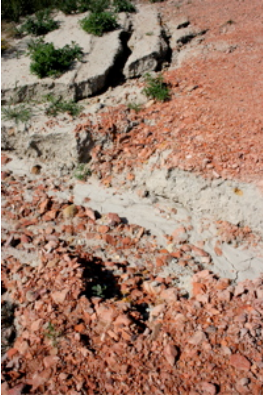
Close-up of crushed clinker used for road-bed materials above bentonite soils on Montana Route 216 about five miles south of Sydney.
