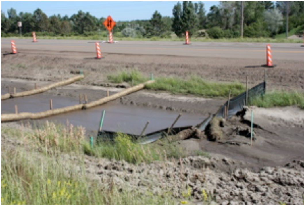
Failed sediment control in the ditch for Route 1804, south of Bismarck, on the afternoon of July 15, 2009.
