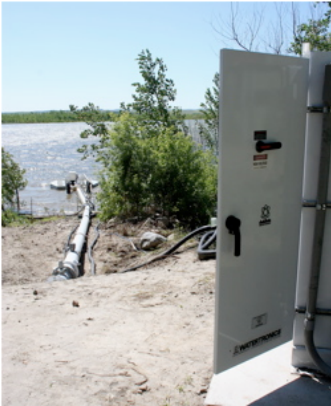
Water pump at lake Oahe, North Dakota.
