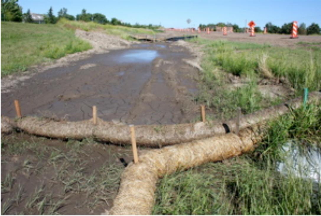
Detail of failed sediment control on Route 1804 south of Bismarck on July 15, 2009.
