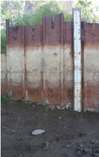
Staff gauge for measuring water height at the Missouri River Bridge at Culbertson, Montana.
