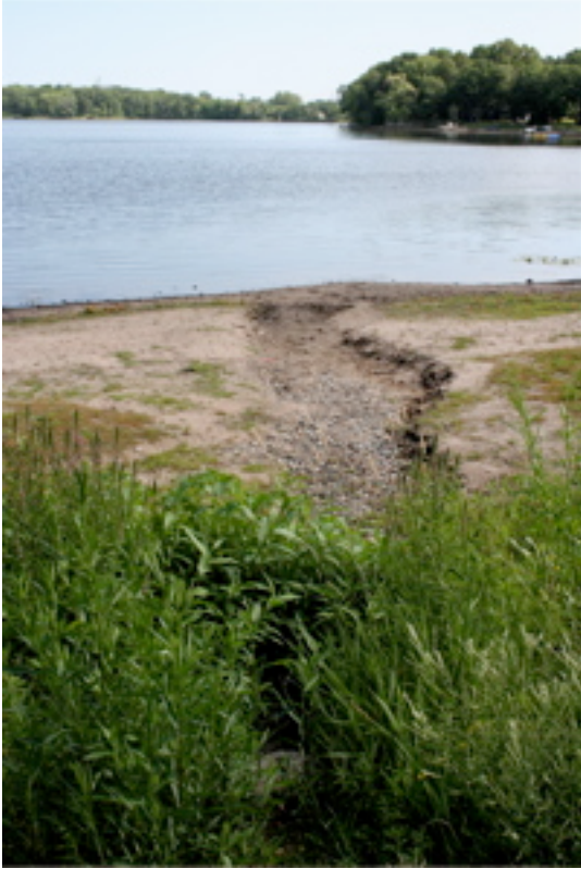
Storm drain entering Silver Lake, North Saint Paul, Minnesota. Not a good idea.
