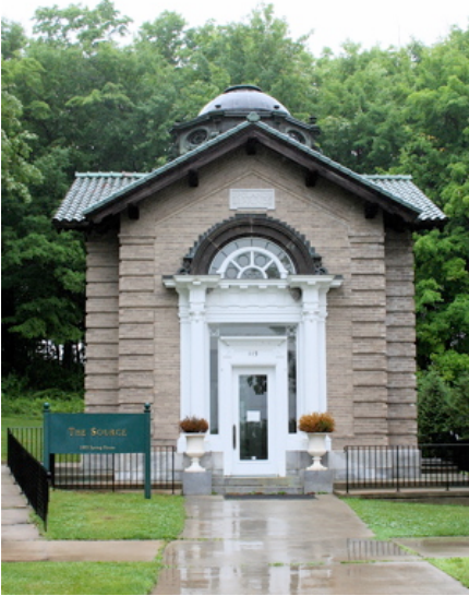
Springhouse at Poland Spring Preservation Park, labeled "The Source."
