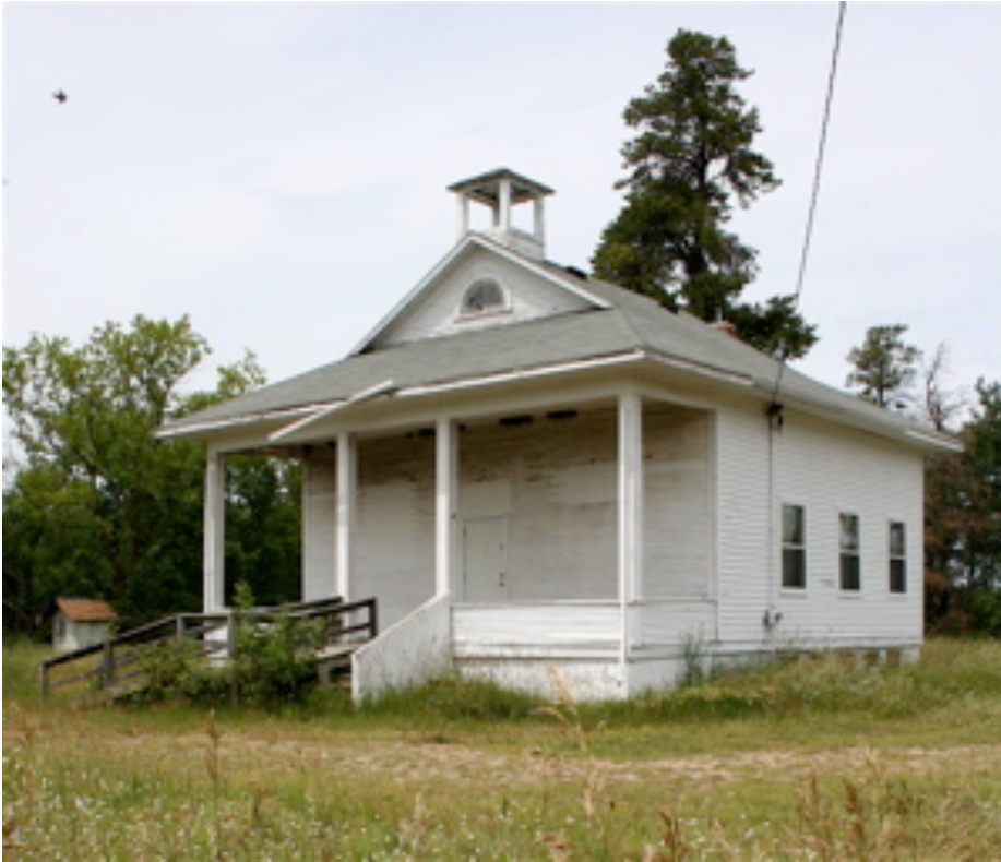
Abandoned building along Route 64 in Poplar, Minnesota.
