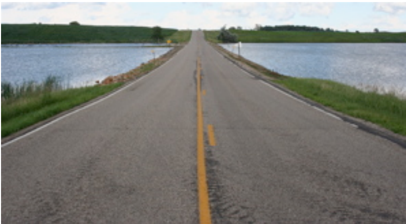
Pothole filled with crushed rock to allow the road to continue in a straight line.
