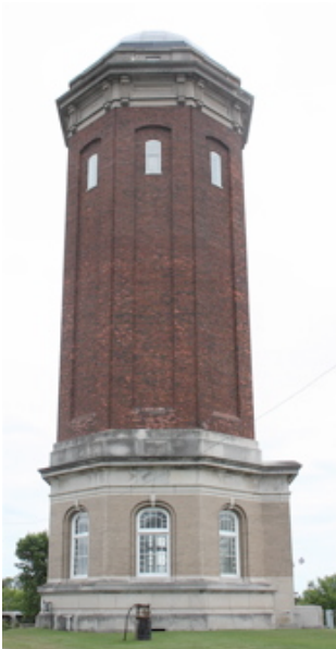
Historic Water Tower in Manistique, Michigan.
