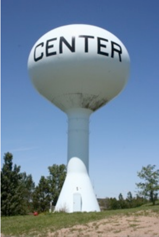
Water tower for Center, North Dakota.
