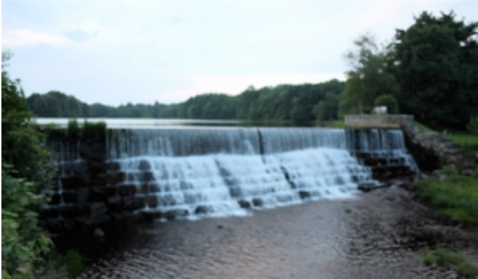
Milldam in Harrisville, RI, built of enormous cut granite stones.
