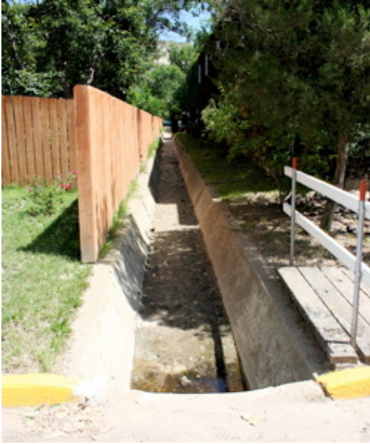
Cement drain in downtown Medora, North Dakota.
