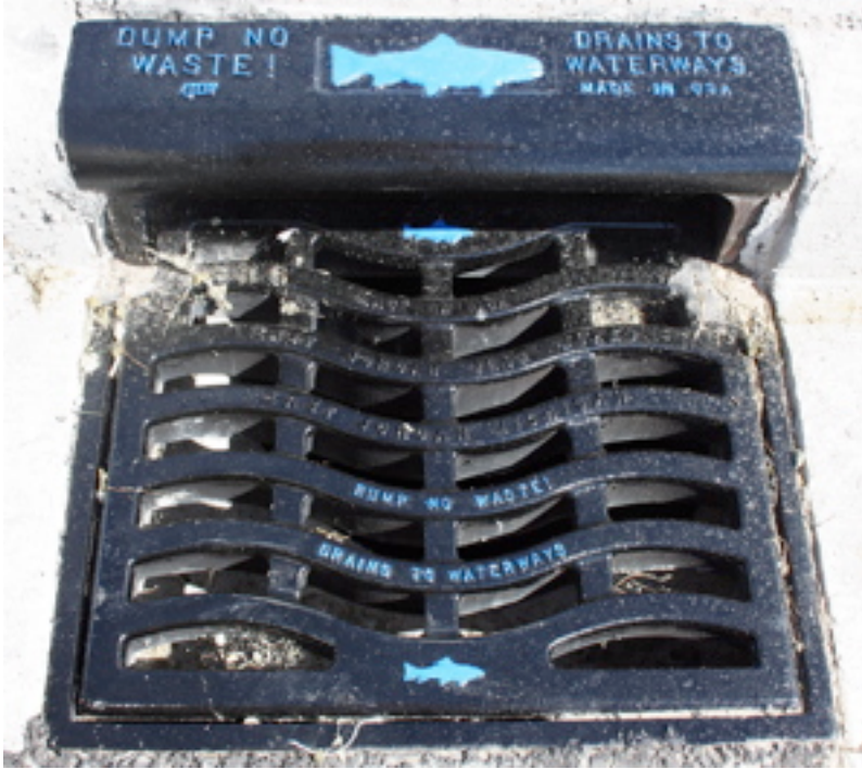
Message on drain at the city pier in Mackinaw City, Michigan, posted directly above the water.
