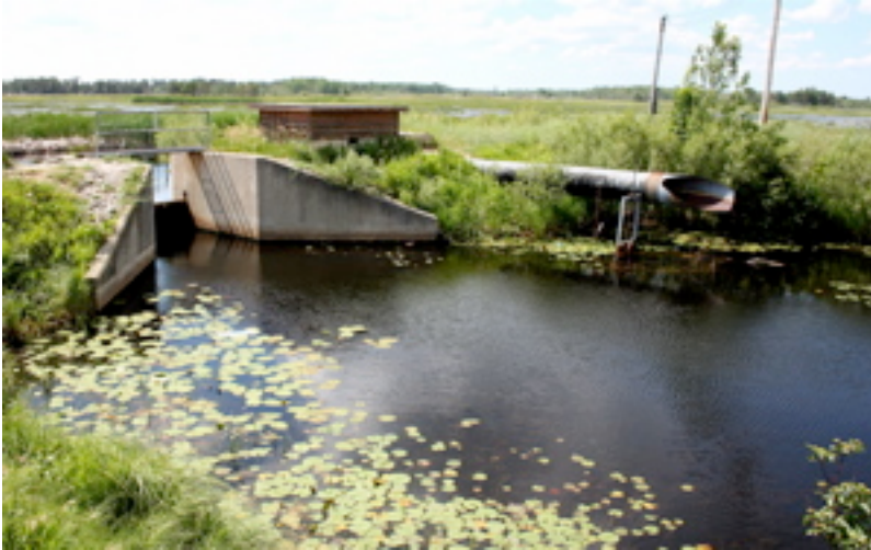
Water control structures for maintained marsh at Houghton Lake Michigan.
