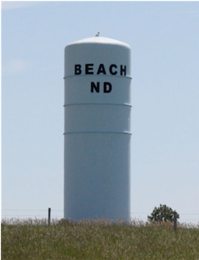
Water tower in Beach, North Dakota, just east of the Montana line.
